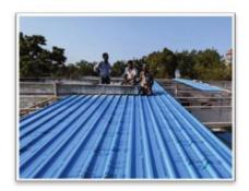
This iron sheet fixing system is very common for the flat roof buildings when they face water leakage problems. This not only reduces the expenditure but also provides safety for the residents, protects the roof from the rain and scorching sun, reduces the summer heat inside the building.
