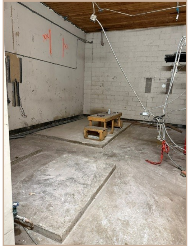
Mechanical room after HVAC removal.
