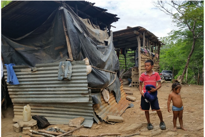
Before: A shack made of tin and plastic held together with a rope is home to a family with six children.
