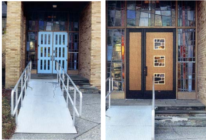
North Doors Before and After Renovations
