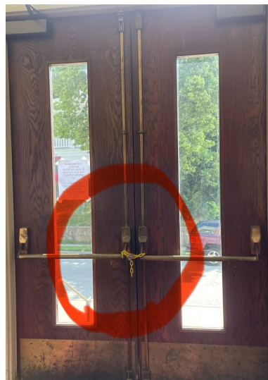
Entrance doors to be replaced
