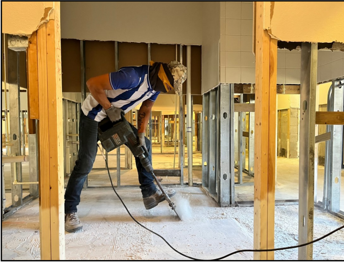
Photos of Construction on 3/3/23. Left: Removal of old tile adhesive in the villas to prepare for new floors. (All the floors were destroyed by post-hurricane flooding.) Right: Removal of concrete in shower stalls prior to drain replacement.
