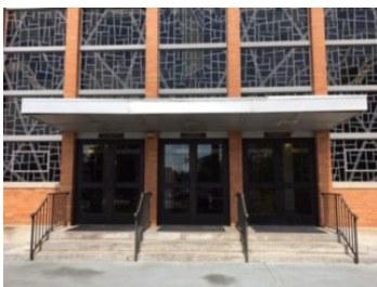
The front porch awning leaks onto the stairs in front of the far right door.
