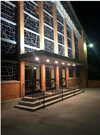
Left side of awning
