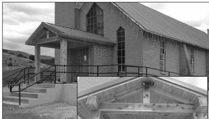
The newly constructed ramp at Our Lady of Guadalupe Mission in Bent.
