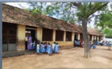
The school buildings in 2018
