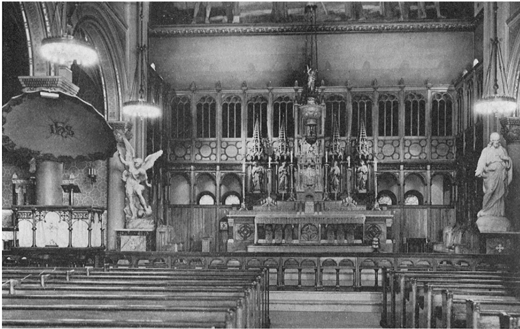
Main Altar before renovation.
