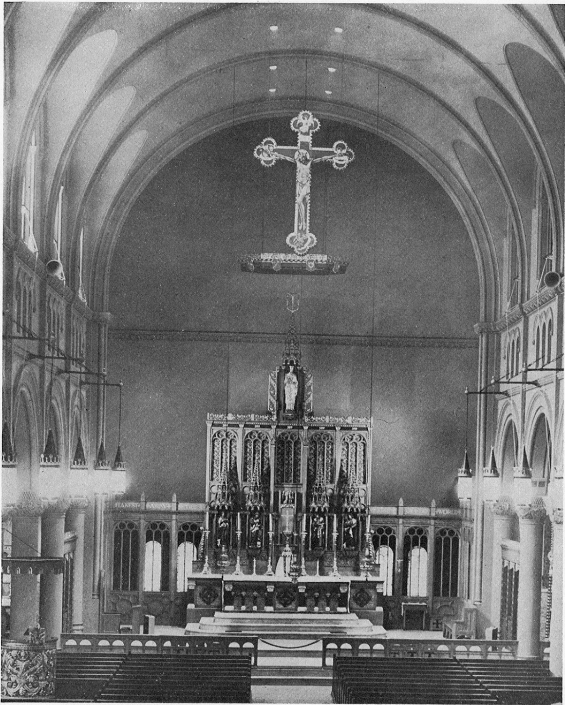
Interior of Church after Renovation
