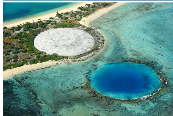
Aerial view of "The Tomb", a concrete covered crater on Runit Island (Photo by Asahi Shimbun/Getty)
