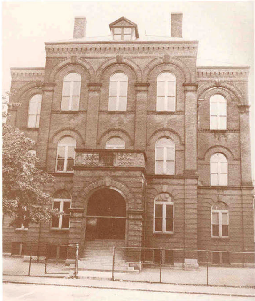
St. John's school, built by Monsignor Thomas Griffin in 1892, stood on Temple Street until it was demolished in 1977. Courtesy Catholic Free Press
