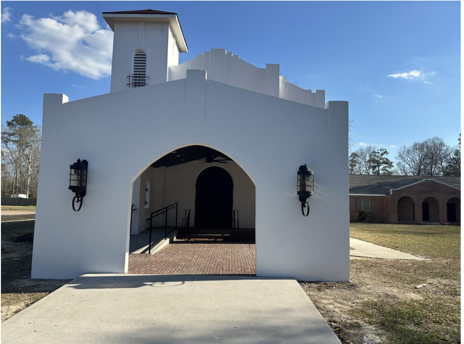
Reconstructed original Portico with Improvements
