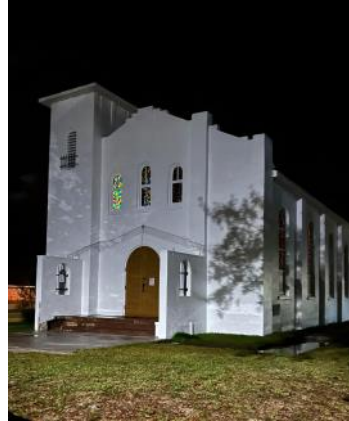
Portico had to be Removed due to termite damage
