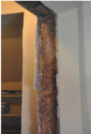
Picture of termite damage
