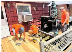
▲ Divine Grace parishioners Ron Hassen, left, and Anthony DiBuono, center, install new decking
