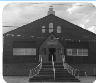
La Asuncion 777 Cortlandt Street Main Office/Oficina Principal
