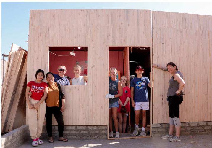
The St. Aloysius team builds a home in Chimbote. (Friends of Chimbote)
