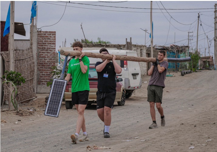
Volunteers on the St. Charles Borromeo team erect a street light in Cambio Puente (Friends of Chimbote)
