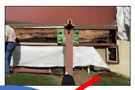
PILE OF ROTTED WOOD FROM THE GLULAM BEAM
