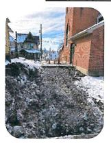
Thanks to some fair weather our construction team did a little demolition. A section of the ramp was broken up, and it will be repurposed. It will be used as back-fill for the block area below the floor of the handicapped access restroom.
