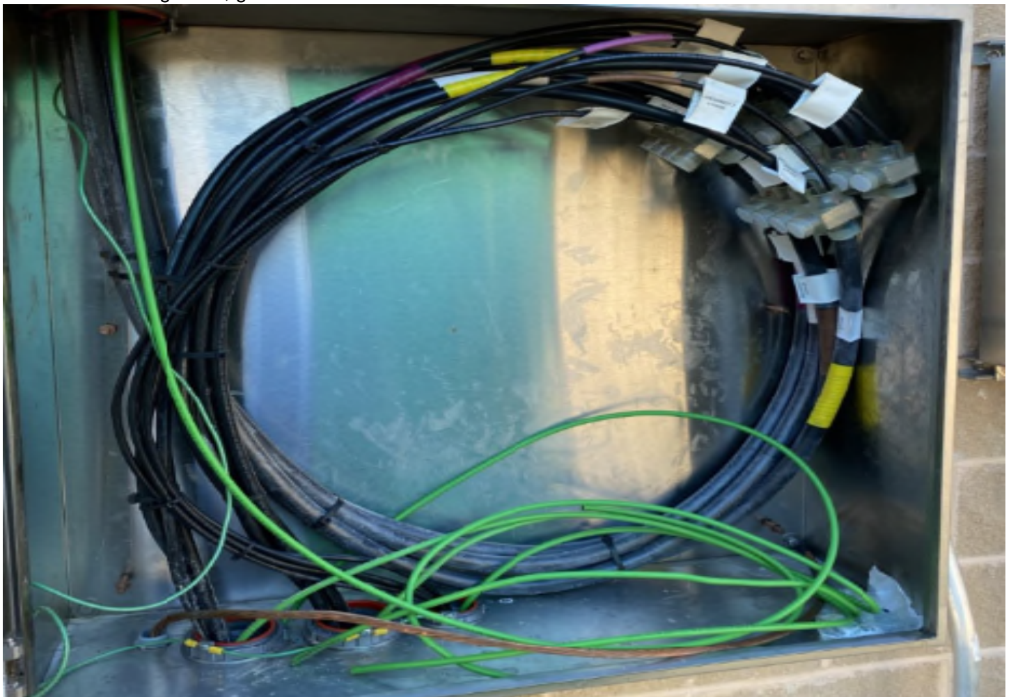
Generator – wiring issue, ground wire not connected
