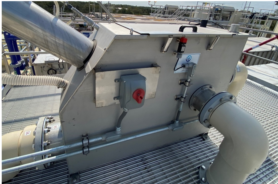
Figure 1. Recently Installed Influent Screen
