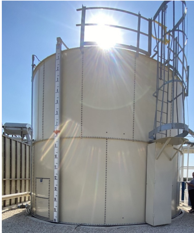
Figure 2. Recently Installed Equalization Tank
