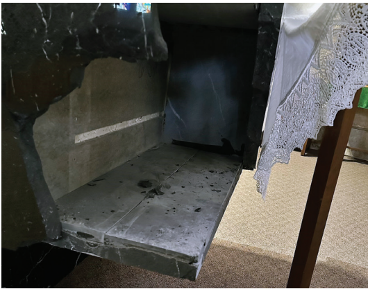
Pictured above is the corner on the original altar where the marble fell off. Photo courtesy of Tom Redle and Julie Este
