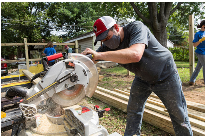
Rich Nigro, with St. Stephen Protomartyr Parish's Holy Name Society, and other workers organized by St. Joseph Housing construct a backyard fence Saturday at a house on Mount Pleasant Street in south St. Louis. Photo Credit: Jerry Naunheim Jr.
