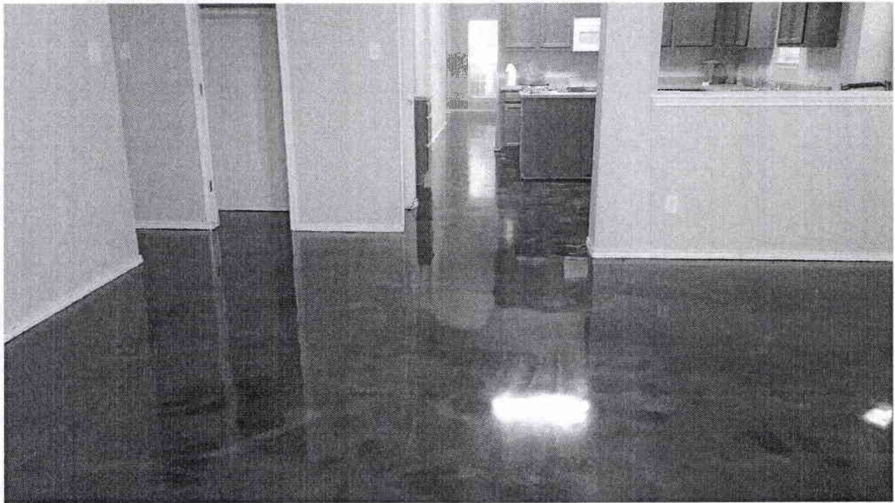
METALLIC EPOXY FLOOR (Color - Chocolate & Copper Kettle)
