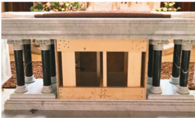
Temporary bracing system under the Altar
