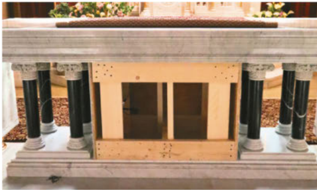
Temporary bracing system under the Altar
