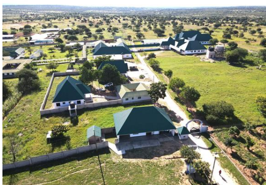
Overhead photo of the impressive building progress at INUKA thanks to HFT donations
