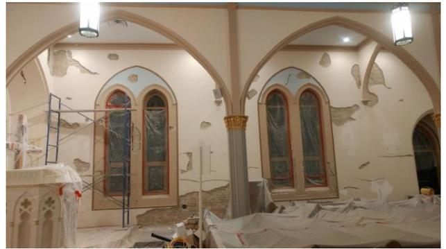
After the roof repairs, the tuck-pointing of the brick structure and the work done on the stained glass windows in the Summer and Fall of last year, the repair work has now entered its second phase. Work now has begun in the interior of the building. As you can see from the pictures, what appeared on the surface to be mere cracks in the walls have turned out to be more than that. The mortar is disintegrating after so many years.
