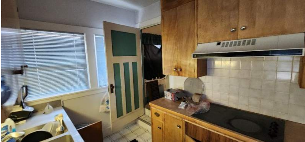
The kitchen has a split stair entry from stairway to the upper level. One stair remains visible on the kitchen side when closed, which is a hazard and not compliant with current codes.
