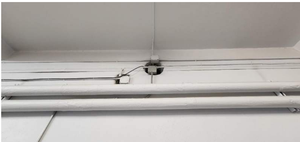
Where previous equipment was removed, holes remain and are used to route utilities through. The above was where a projector once shone through.
