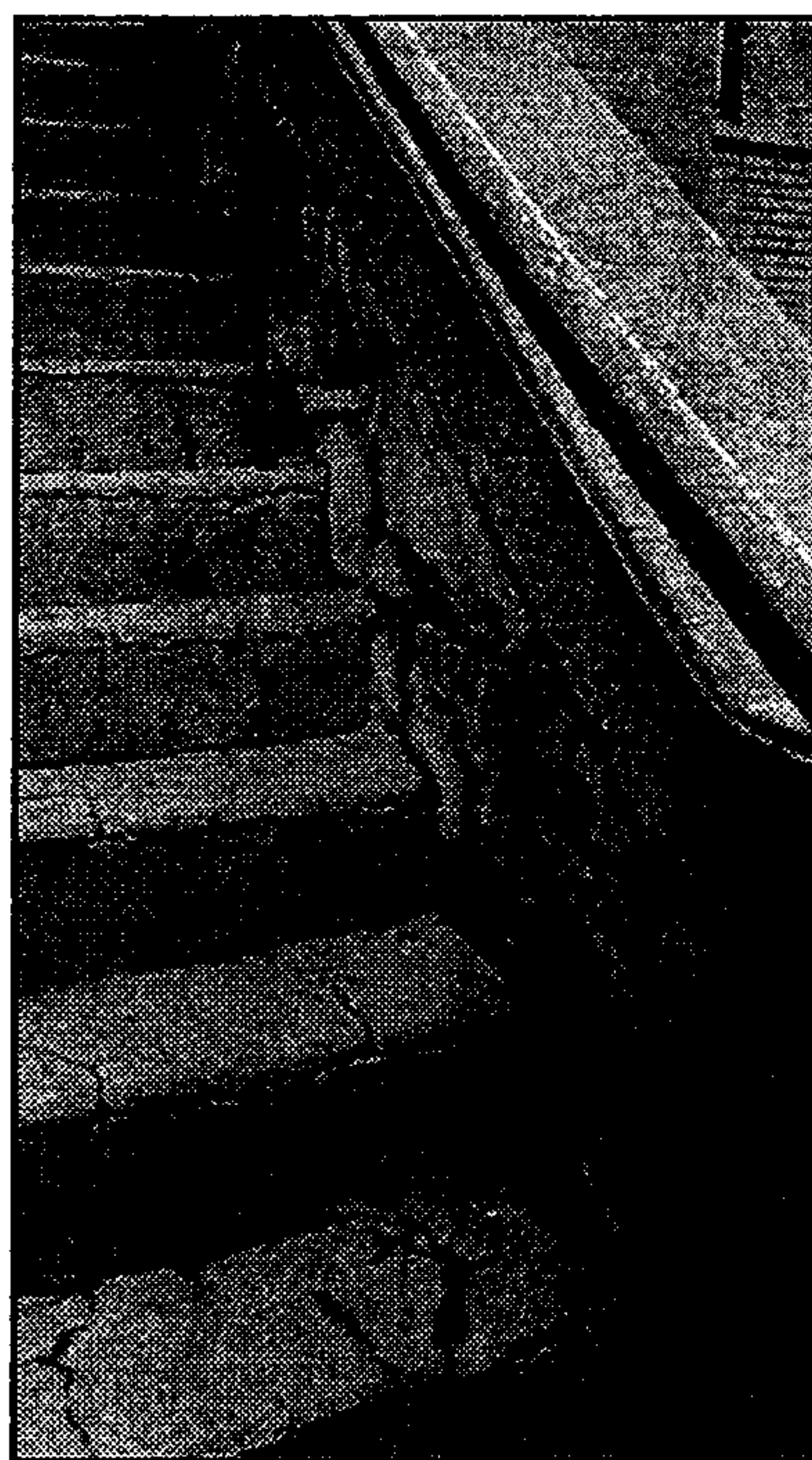
Note: Deterioration of concrete and sandstone.
