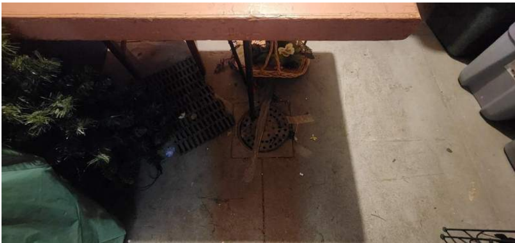
Floor drains are present in the larger storage area.
