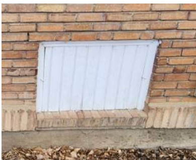
Various windows have been infilled
