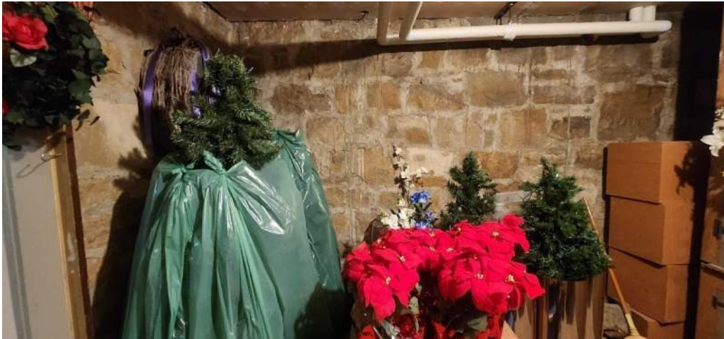
The small portions of the building remain with a sandstone foundation or load bearing wall. Toward the south and under the main entry stair, some water staining was visible on the stones. No excessive wear is visible and the stones remain in good condition.
