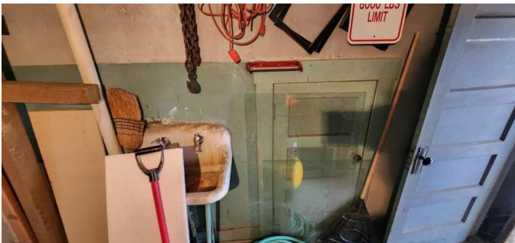
A smaller door to access space under the exterior stair to the sanctuary above, not opened.
