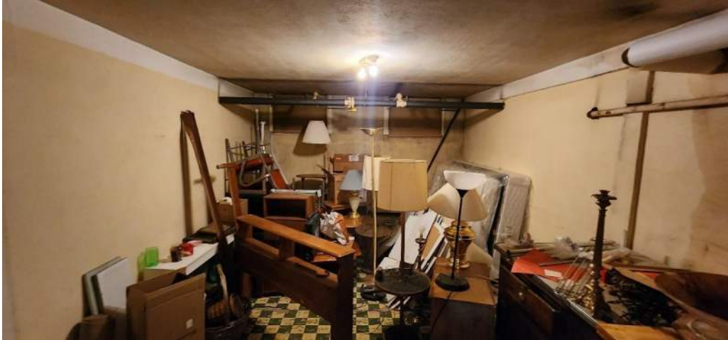
Various plumbing pipes are routed through the spaces below, some in a fashion that appears to be from retrofit work at some point as they are placed sporadically.
