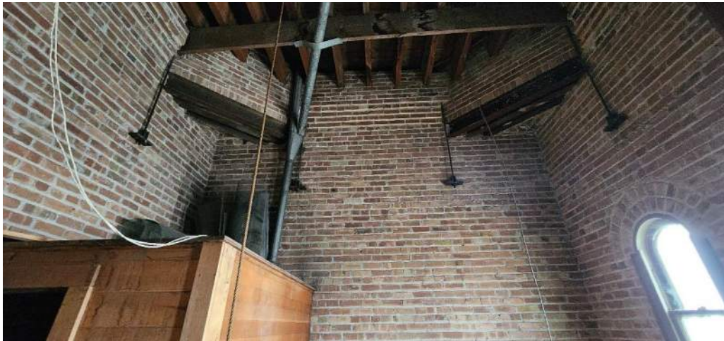
Brick in the upper Belfry appears in good condition. Structural connections for the main belltower above appear in good condition.
