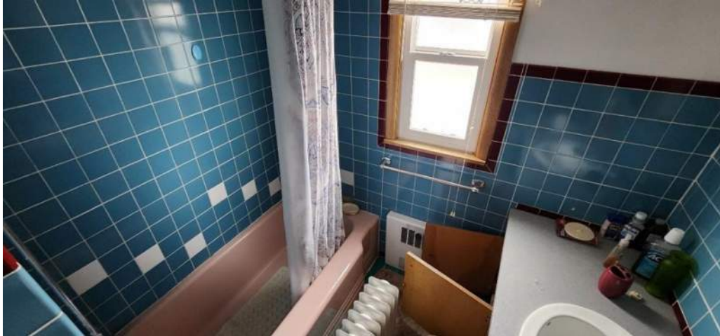
Wall tiling in the bathroom is in good condition. The flooring is aged. Fixtures are original.
