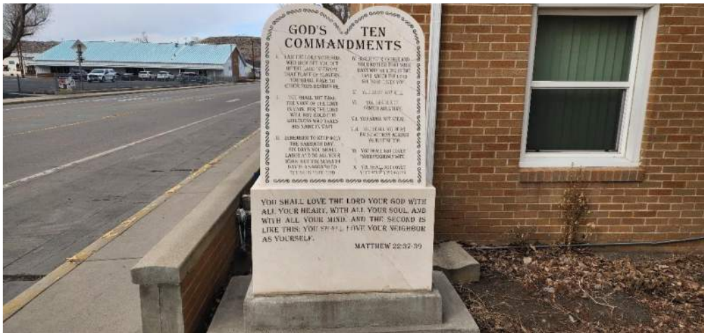
Ten commandments are on display. Stone is cracked and should be repaired/replaced. The base shows signs of weather, but is not failing.
