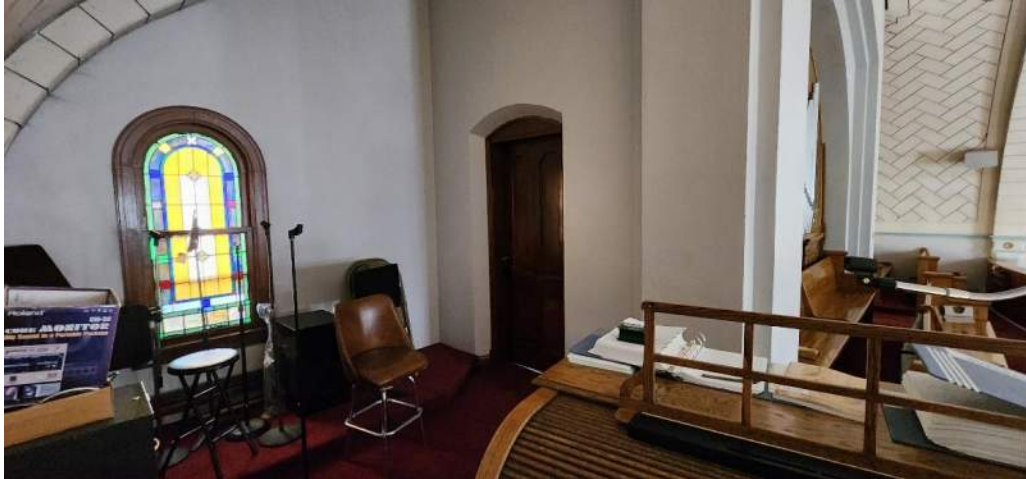
Another access point to the Belfry exists on the balcony. As noted elsewhere, safe egress is compromised from within the Belfry.
