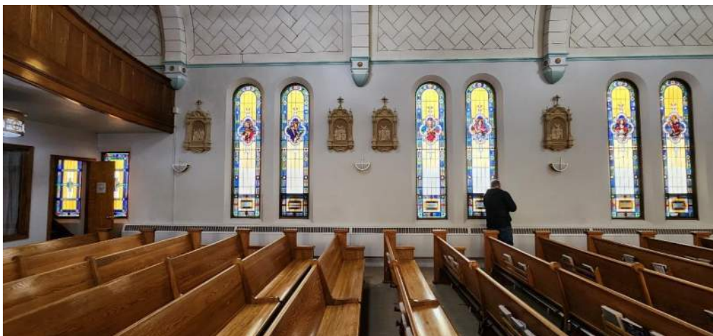
Stained glass is present on the interior, storm windows are present to protect them on the exterior.
