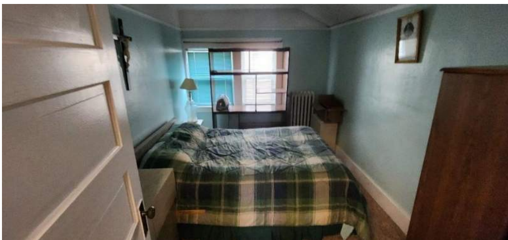
Doors throughout appear to all be original and in satisfactory condition.
