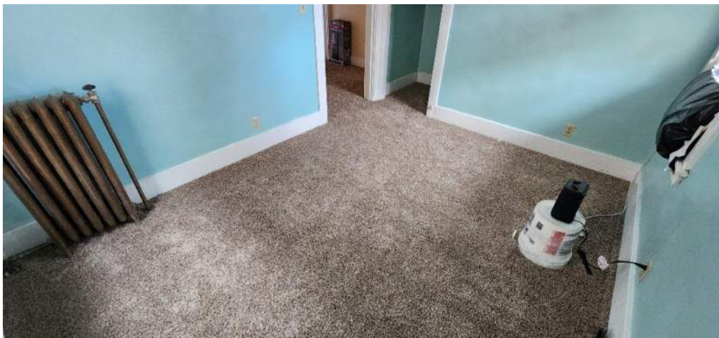
Carpet was clean and taut. No flooring concerns noted.
