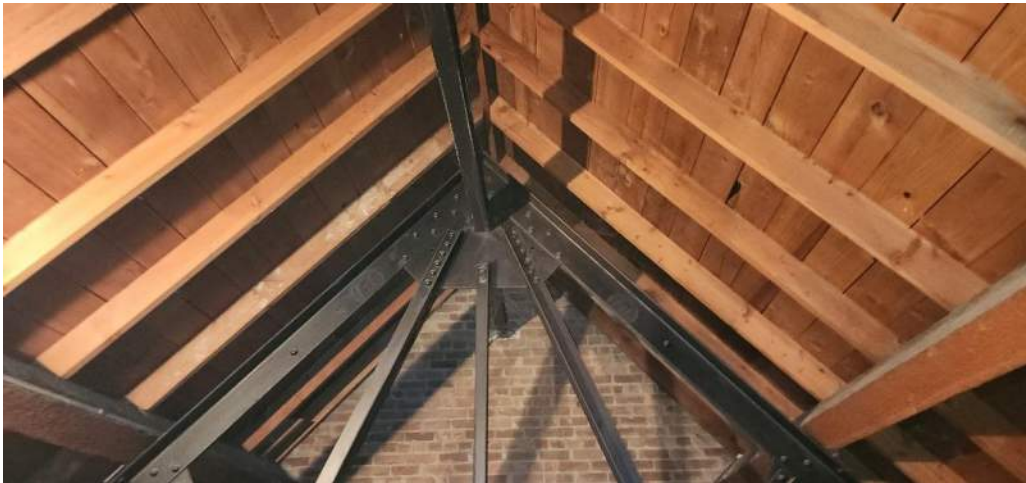
Steel structure remains without issue, no signs of fatigue, rust, or otherwise visible.
