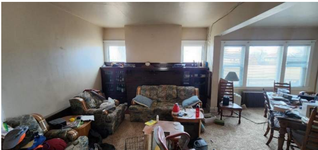
An old fireplace has been filled in, the mantle and casework around it remain.
