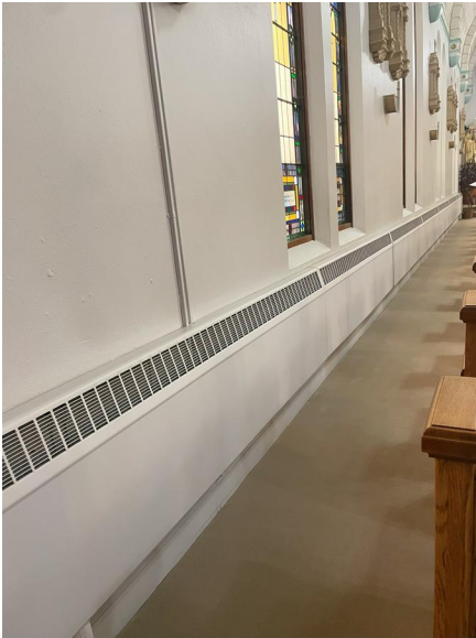
Perimeter Finned Tube Radiation
