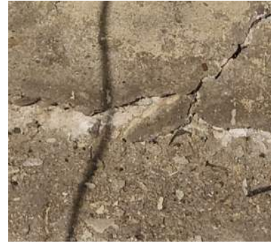
Concrete cracking/spalling
