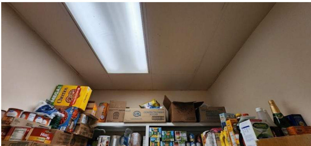
Items are stored within 18" of a ceiling, non-compliant with the International Fire Code, Chapter 3.
