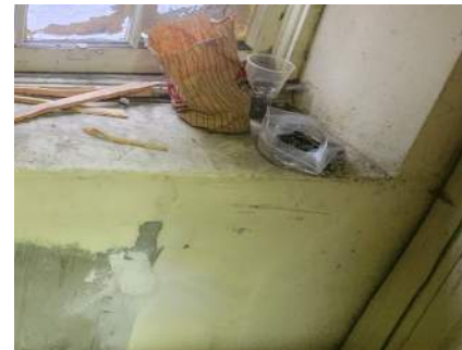
Sound concrete window sill
