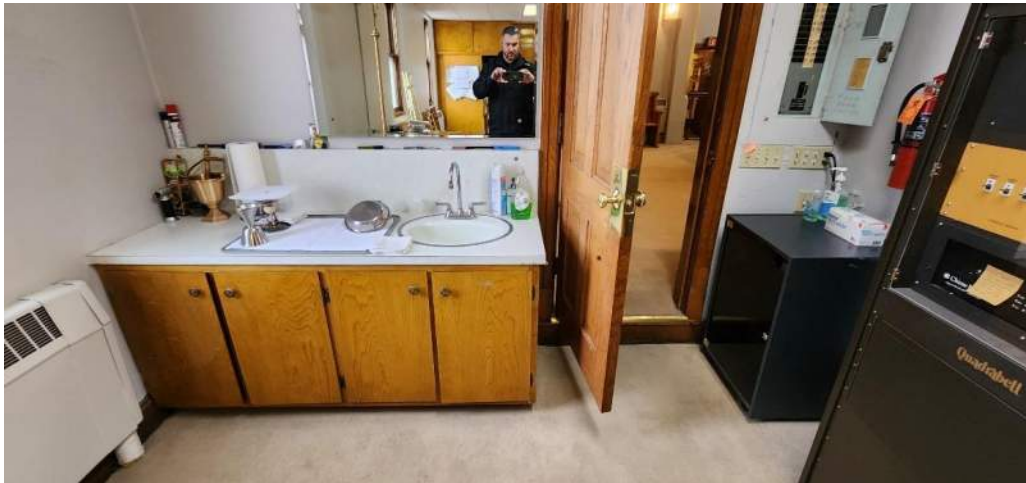
The Sacristy contains plumbing and electronics for music and bells. The space appears to be in overall good condition. A level room-to-room transition would allow for barrier free access.
