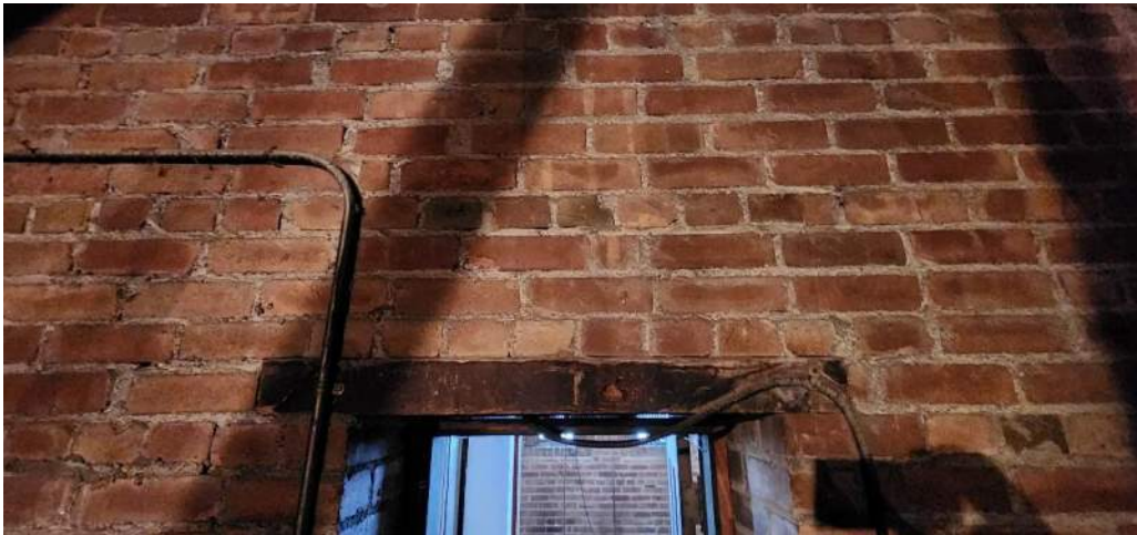
Brick visible within the catwalk appears to be in good condition. Old electrical is visible, with new conduit having been installed for attic access lighting.
