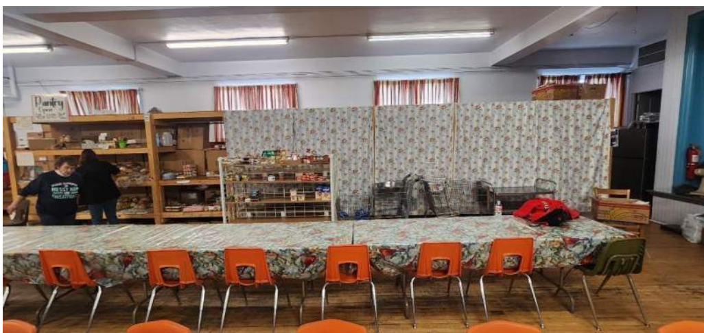
The floor is worn and requires repair for sanitary use within an eating establishment. A pantry and dry storage area are designated with. The space has been adapted by any means to provide the services of a soup kitchen.
