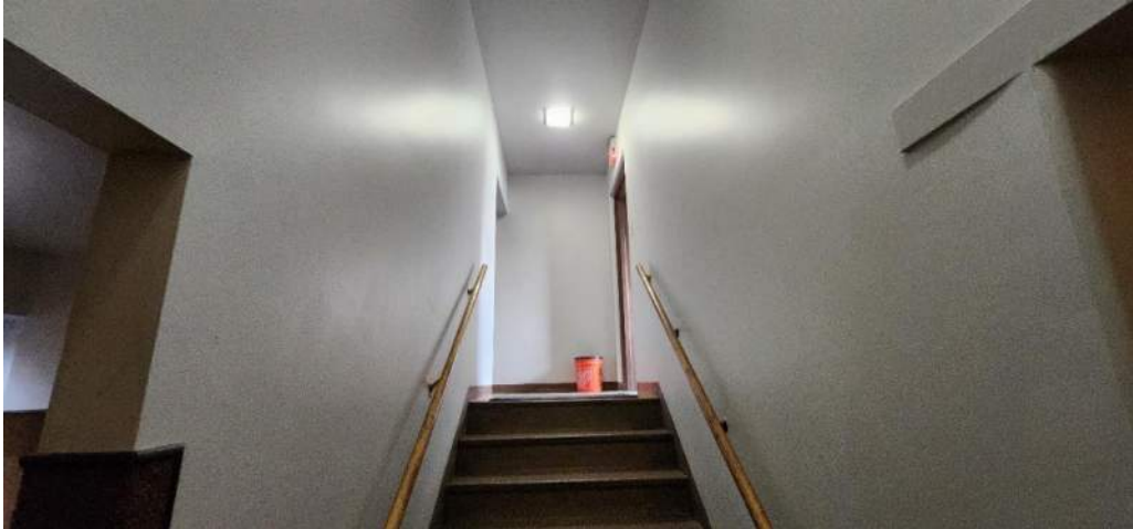
Landings and stair widths are adequate in the addition to be considered for path of egress.
