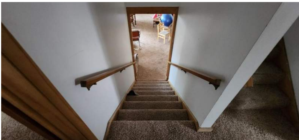
Carpet throughout was in decent condition and has been replaced in the past. Stairs have hand rails on both sides and comply with residential requirements.
