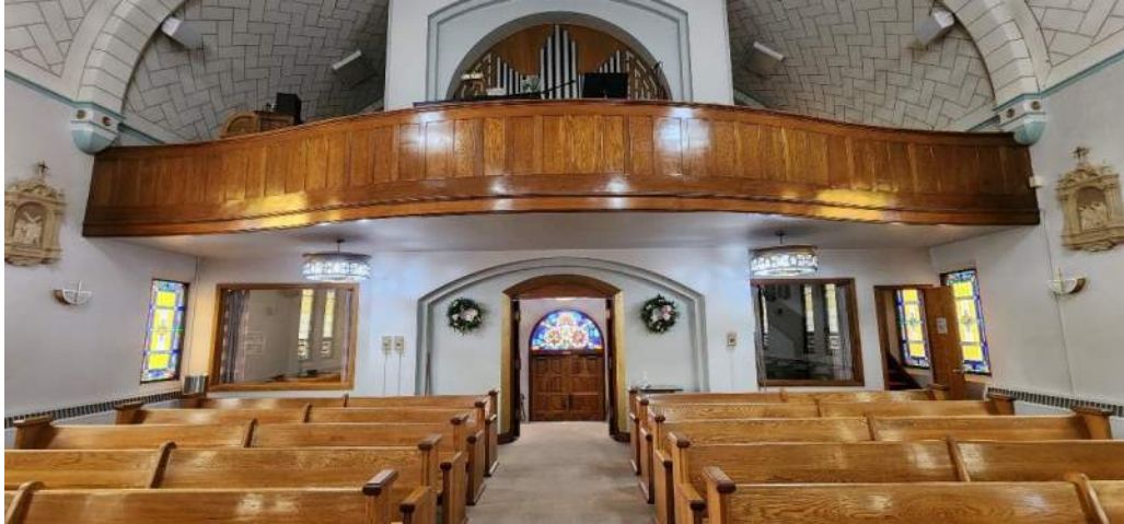
The Choir and Organ balcony is also well maintained. Narrow stairs are present for able body access, no means for disability access exists to the balcony, limiting its use.
