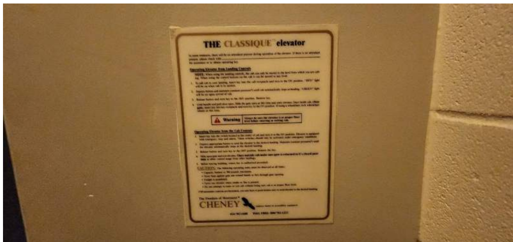
The elevator is considered "Limited Use/Limited Access" (LULA) under the current building codes. Meaning it is allowed to a component of the accessible route, but has limitations. This unit does not have an automatic return to floor function upon loss of power, leaving users stranded.
