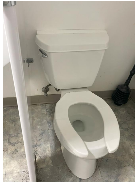
Basement Main Bathroom Typical Fixture
