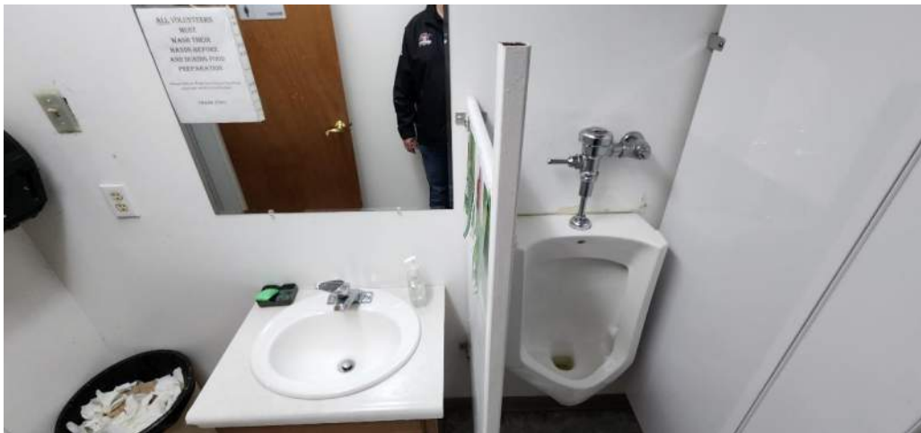
There is a larger toilet room with both urinal and toilet stall. Again the hard and non-absorbent finishes around fixtures as outlined in the International Building Code.
