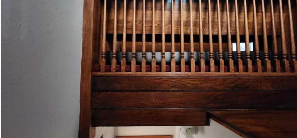
The Choir Balcony has compliant guard rail construction with properly spaced balusters present.
