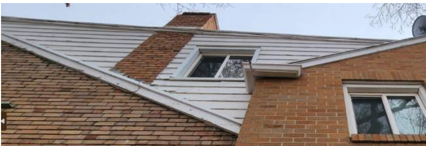
Infill construction between original Rectory and Offices
