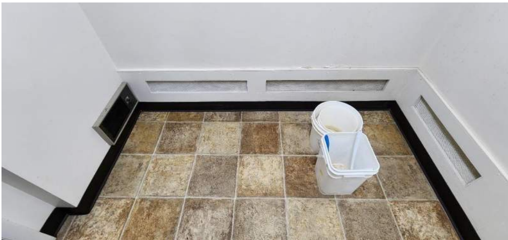
Ventilated cavities are present in the base of the wall on 2 sides. Use of these is unknown. It is believed these cavities may exist to allow ventilation in the walls to mitigate moisture infiltration.
