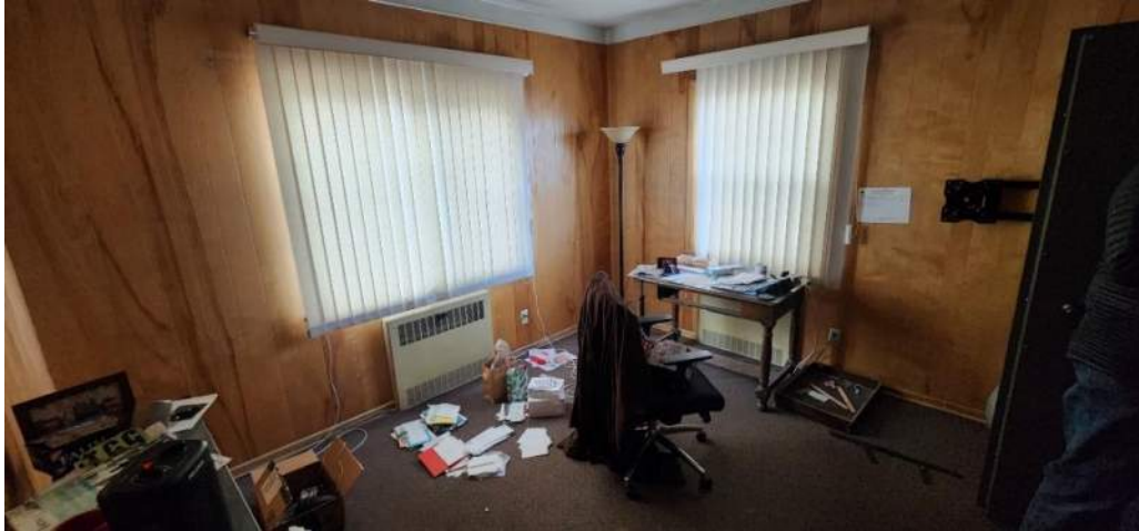
Finishes are aged but do not show significant failures or signs of potential failure.
