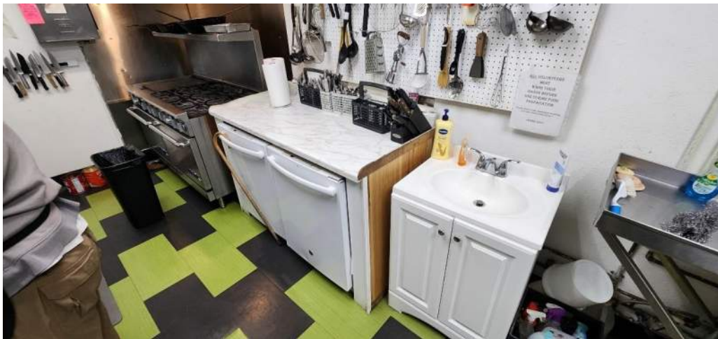
The kitchen has bare minimums for compliance, i.e., a suppression hood over the stove and a 3-compartment sink. Other items lack sanitary requirement. I.E. pours wood surfaces or worn laminate on wood. Items should be replaced with stainless food service grade equipment.
