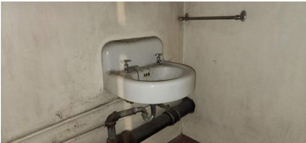
The sink remains intact within the basement.
