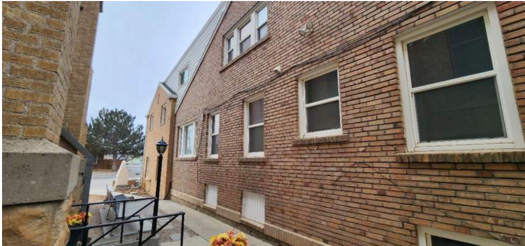
Utilities can be seen anchored to the façade of the Rectory. There is a sidewalk along the foundation, and a permeable surface next to that.
