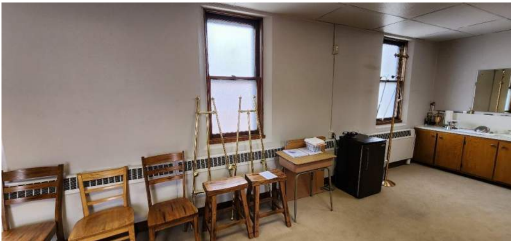
Boiler heat is present in the Sacristy. Windows are operable to allow for fresh air within the space.
