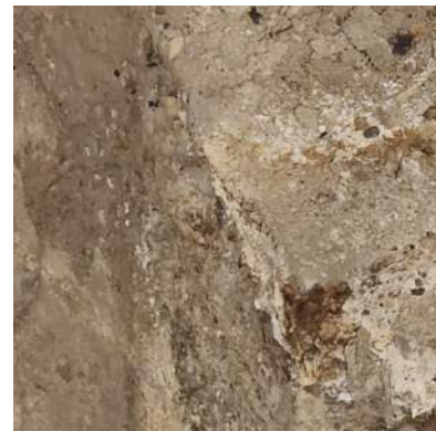
Significant spalling
