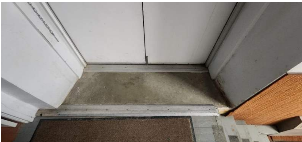
Thresholds were present to provide smooth transitions at the exterior loading/egress door.
