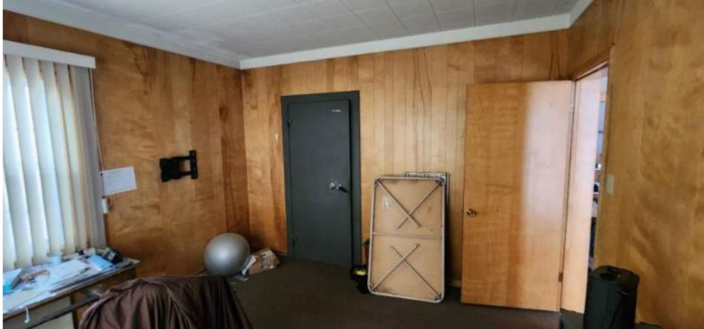
Finishes are aged but do not show significant failures or signs of potential failure. There are signs of previous ceiling repairs made at the exterior wall.
