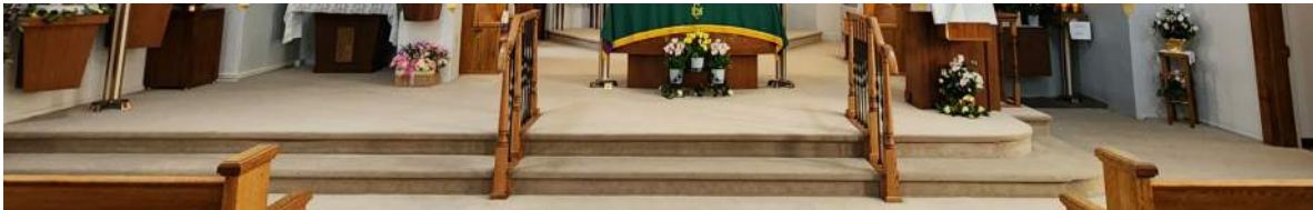
No accessible route to Altar is provided
