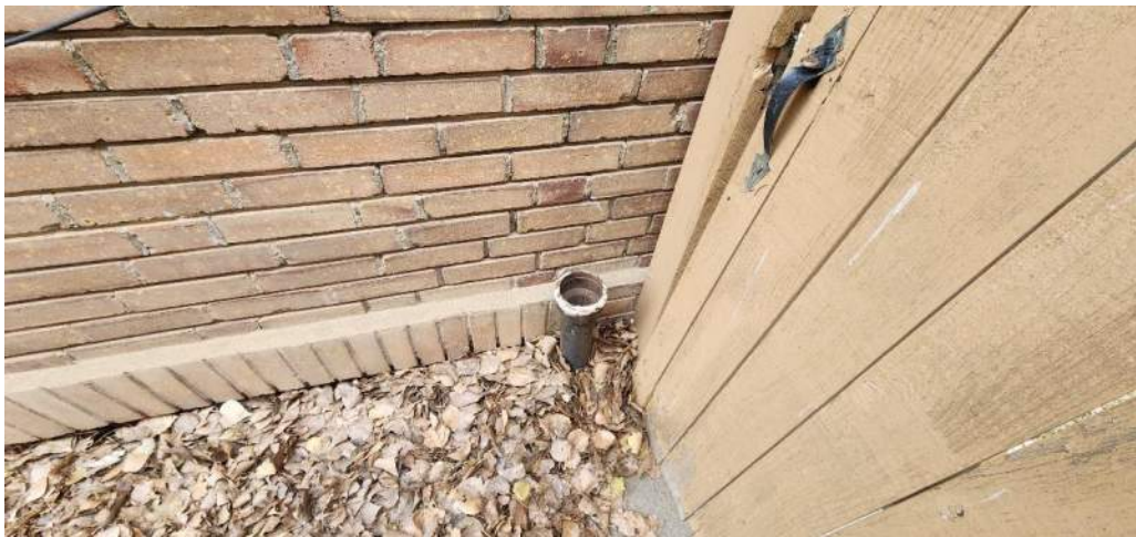
Remnants of what appears to be a test well to monitor moisture in the soil remains. If correct, it was likely used to observe moisture influence of soils on the foundation.
