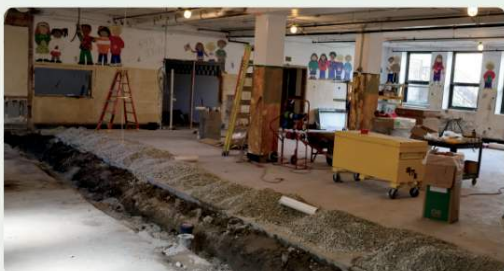
CAFETERIA UNDER CONSTRUCTION
