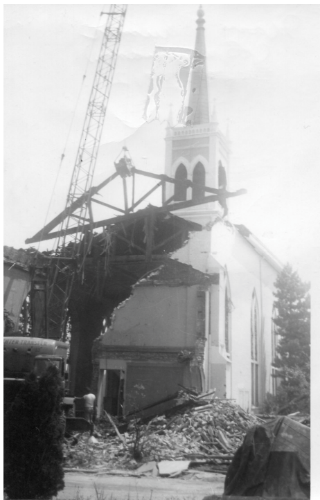
Demolition of the 1849 church
