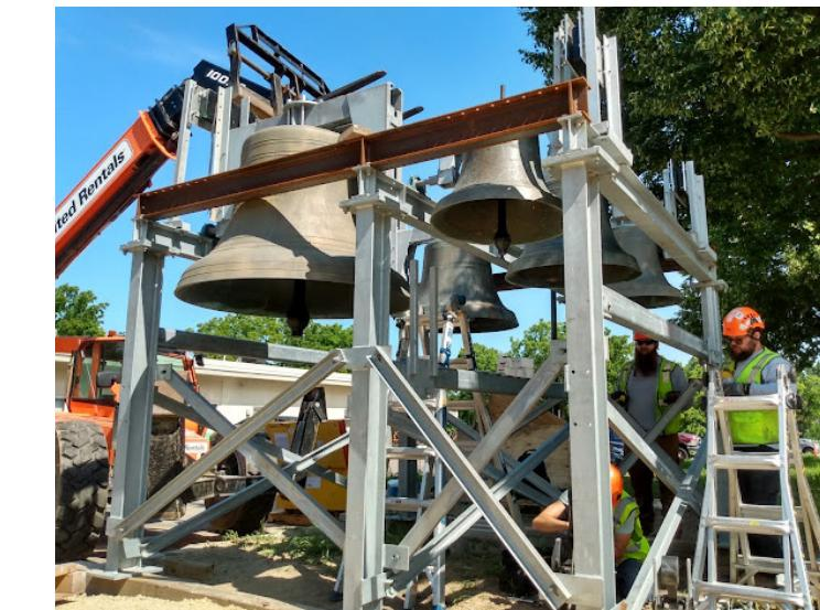
will attach to the inside of the tower. The bells and their framing will fit inside the larger structure. The larger structure is required for the (God willing) installation of the spire. Once the larger structure is prepared, both structures will be lifted by a crane into the tower. We still have a few weeks until that happens, and it will largely depend on weather conditions as cranes are extremely sensitive to wind gusts. Please keep this part of the project in prayer.
