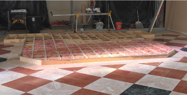
Pictured above is construction of the predella for the main altar and the reredos. Pictured at left is construction of the predella for the bishop’s cathedra.
