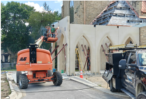
The front fascia of the covered parking lot entrance is welded in place.
