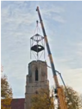
The support structure is prepared to be lowered into the bell tower.
