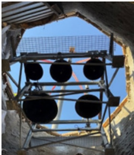
A photo from inside the bell tower as the bells are lowered into place.
