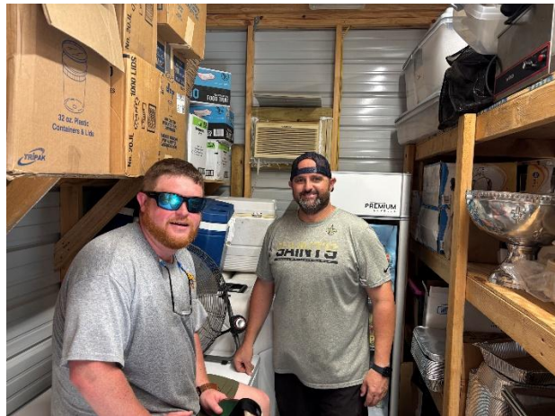
A/C installed in the storage shed
