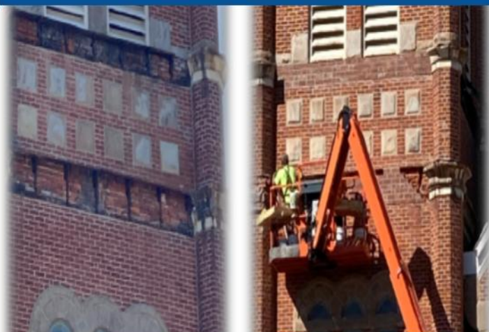
BEFORE—Bricks uncovered under metal sheeting
