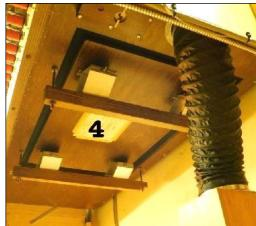
The OLV pipe organ consists of one small blower (¾ horsepower) inside of a box (1). The box is designed to muffle the sound of the blower in operation. There are three small reservoirs (2) and several wind lines constructed of wood (3) and plastic flexible tubing (3).
