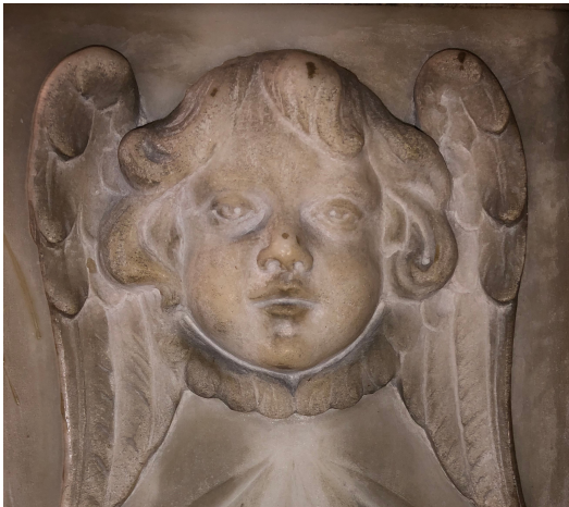
Refabricated and installed 14 missing/fractured decorative stones on the main altar as well as 8 on the side altars.
