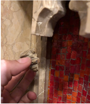
Refabricated and installed 14 missing/fractured decorative stones on the main altar as well as 8 on the side altars.
