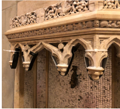
Refabricated and installed 14 missing/fractured decorative stones on the main altar as well as 8 on the side altars.
